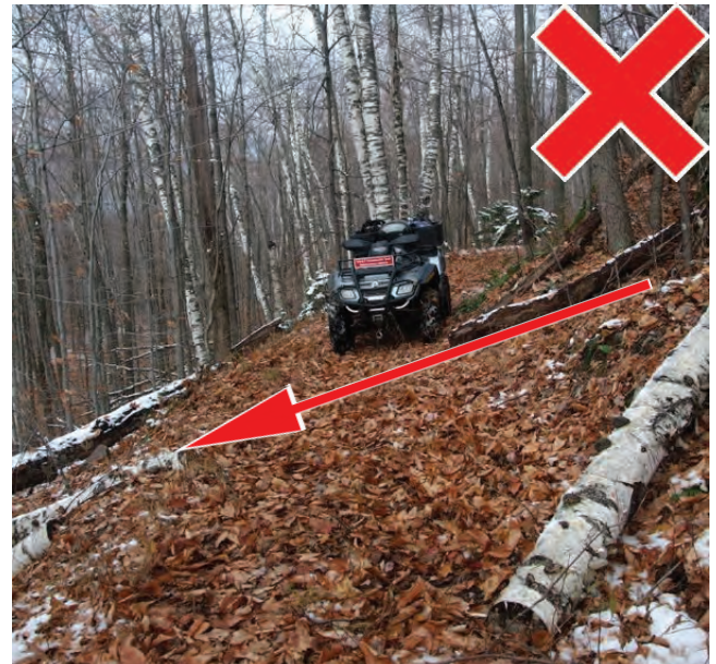
This out-sloped trail can be hazardous for riders and groomers. Never out-slope a trail!
