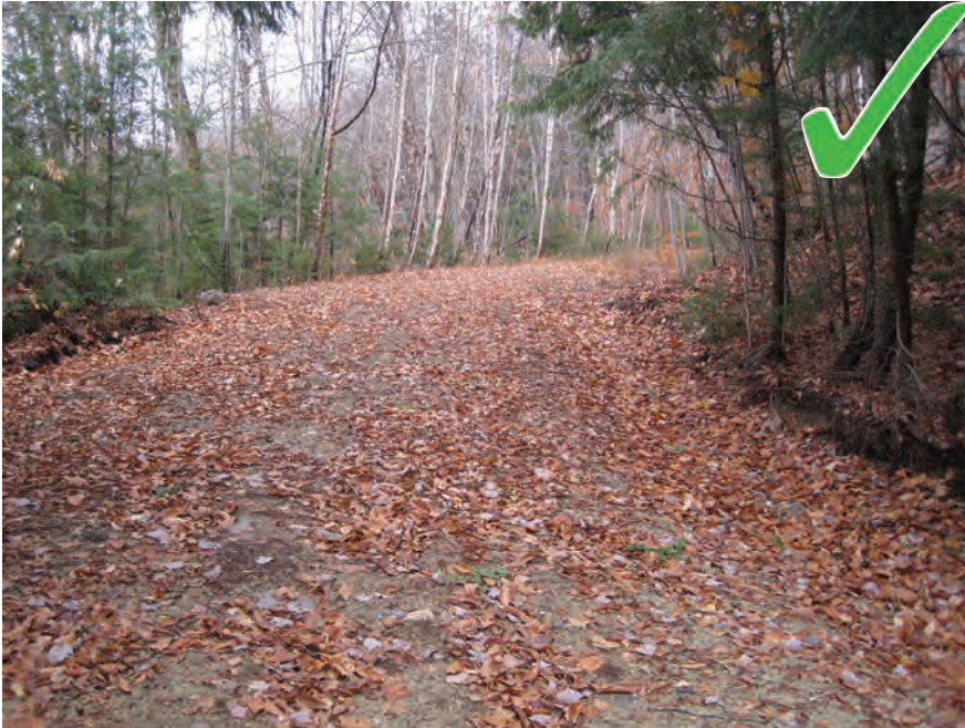
This wide curve will allow riders to safely and comfortably navigate the turn.
