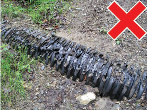
Plastic culverts can be more expensive than metal ones, but they last longer. Because they are much lighter, frost can shift them in the ground easier if they are not covered deep enough with good materials.
