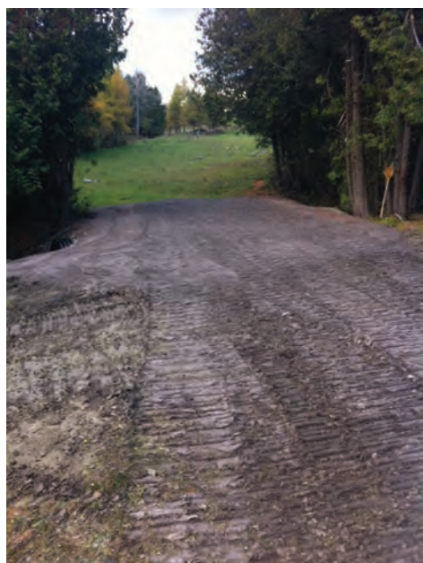
Trails in some areas may need to be reinforced with crushed stone or gravel when native materials are unavailable or of poor quality. This helps elevate the tread and resist erosion. Make sure that you are not adding fill to wetlands, streams, seeps, and vernal pools..
