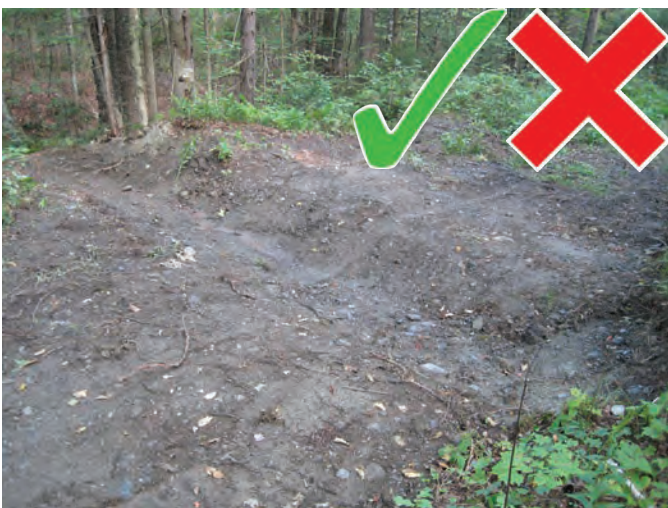
This drain dip will catch water, but should be broadened out for a smoother trail experience. Make sure that your outflow point is lower than the other side of the trail.
