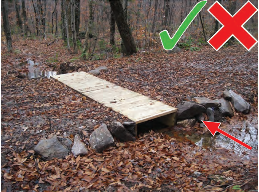
Wooden Box culverts are an inexpensive alternative when flows are small. When placing a culvert, make sure that it is in line with the water flow to prevent a washout.
