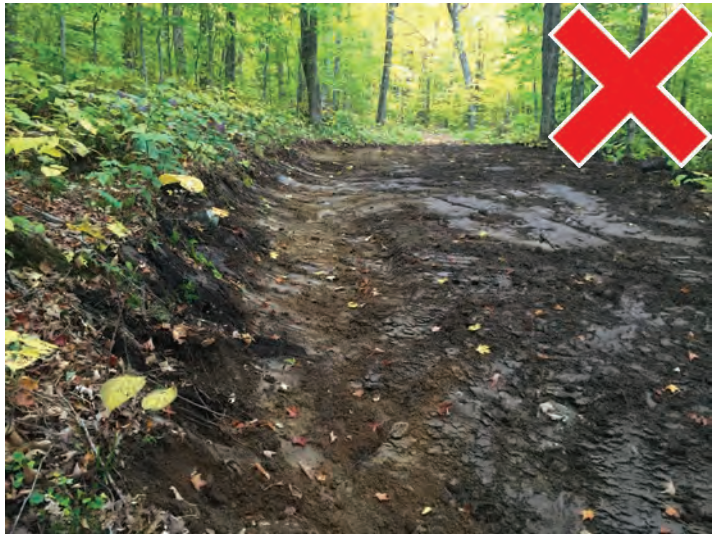
This ditch is far too shallow to control the flow of water. Remember that to move water in a ditch, one end needs to be lower than the other.
