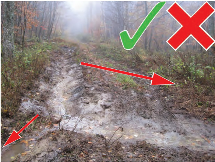
While this is a good example of a drain dip as an outflow, the water is flowing past the dip (bottom left). The tread is sloped away from the ditch instead of towards it.
