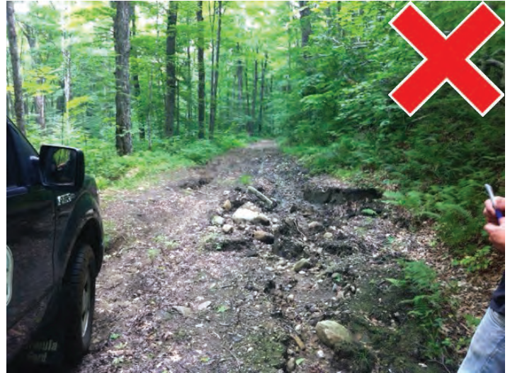
When water cannot flow off trail, it will run down the trail damaging the surface.
