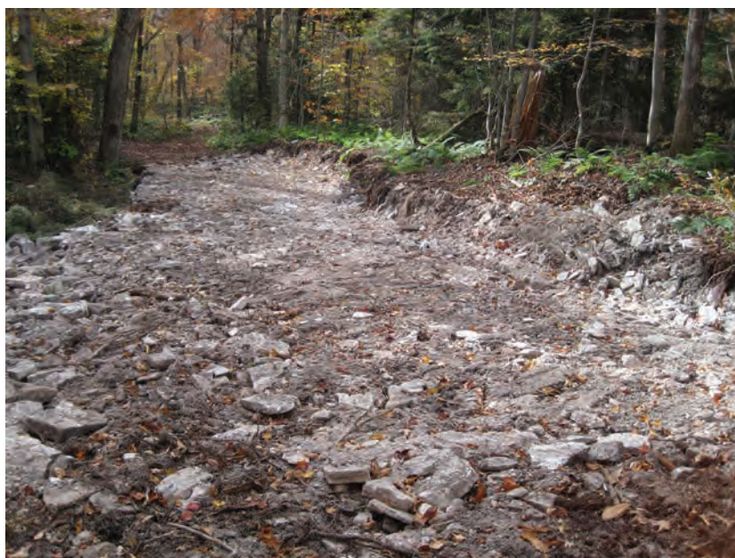
Trails in some areas may need to be reinforced with crushed stone or gravel when native materials are unavailable or of poor quality. This helps elevate the tread and resist erosion. Make sure that you are not adding fill to wetlands, streams, seeps, and vernal pools..
