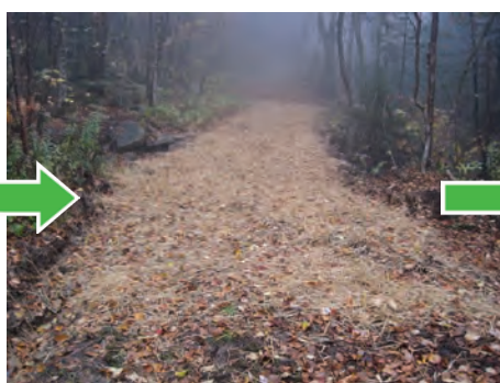
After tread work, give the trail time to set and harden before running equipment or maintenance vehicles on it.
